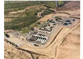
St. George Waste Water Treatment Plant in Bloomington
