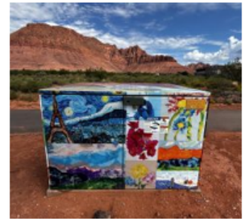
Wrapped utility box at Vista School
