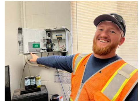
Joseph Rawlinson shows the communication module that allows remote management of the irrigation system at Unity Park.
