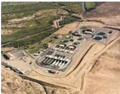
St George Waste Water Treatment Plant in Bloomington
